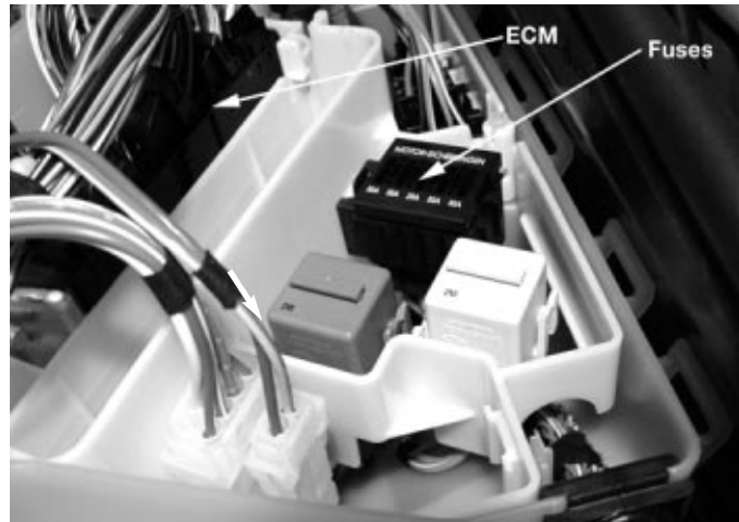
E46 Electronics Box - ECM and Fuses
